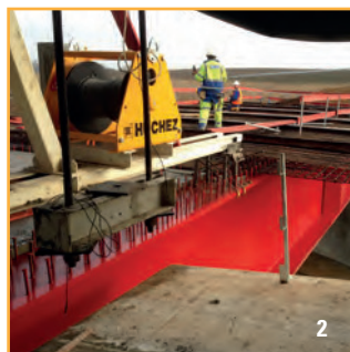
2. Installation of a formwork on a construction site.
